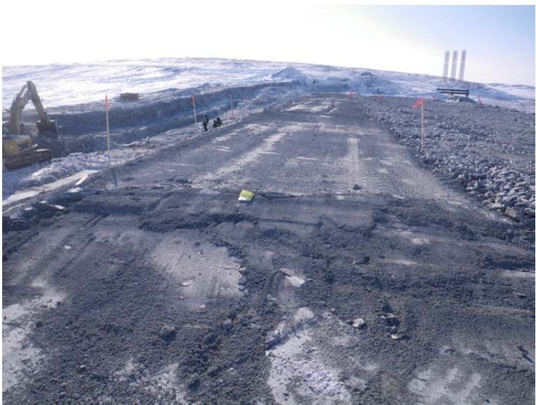
Photo 6: End of FCM placed March 21 nightshift, the end of the placed material was scrapped and removed prior to freeze back.
