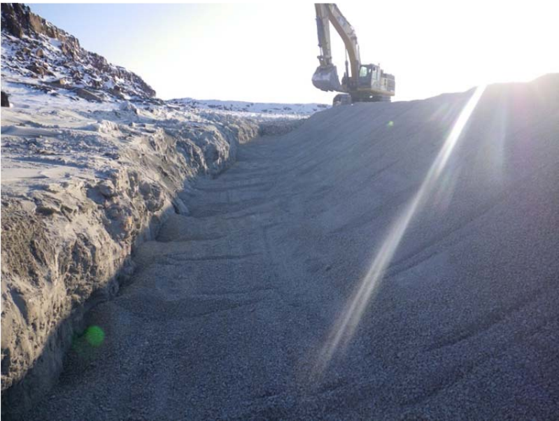
Photo 8: Under liner crush surface at diversion berm. Photo looking east.
