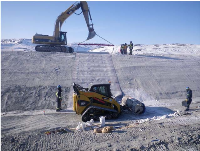
Photo 4: Placing on panel of GCL, skidsteer holding panel at bottom for placement.
