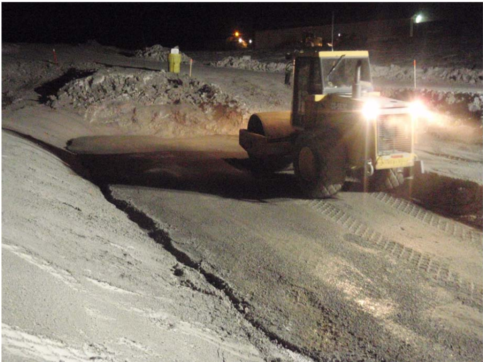
Photo 10: View of vibratory packer on third Overliner lift (1 st today) at the North end of the dam alignment.
