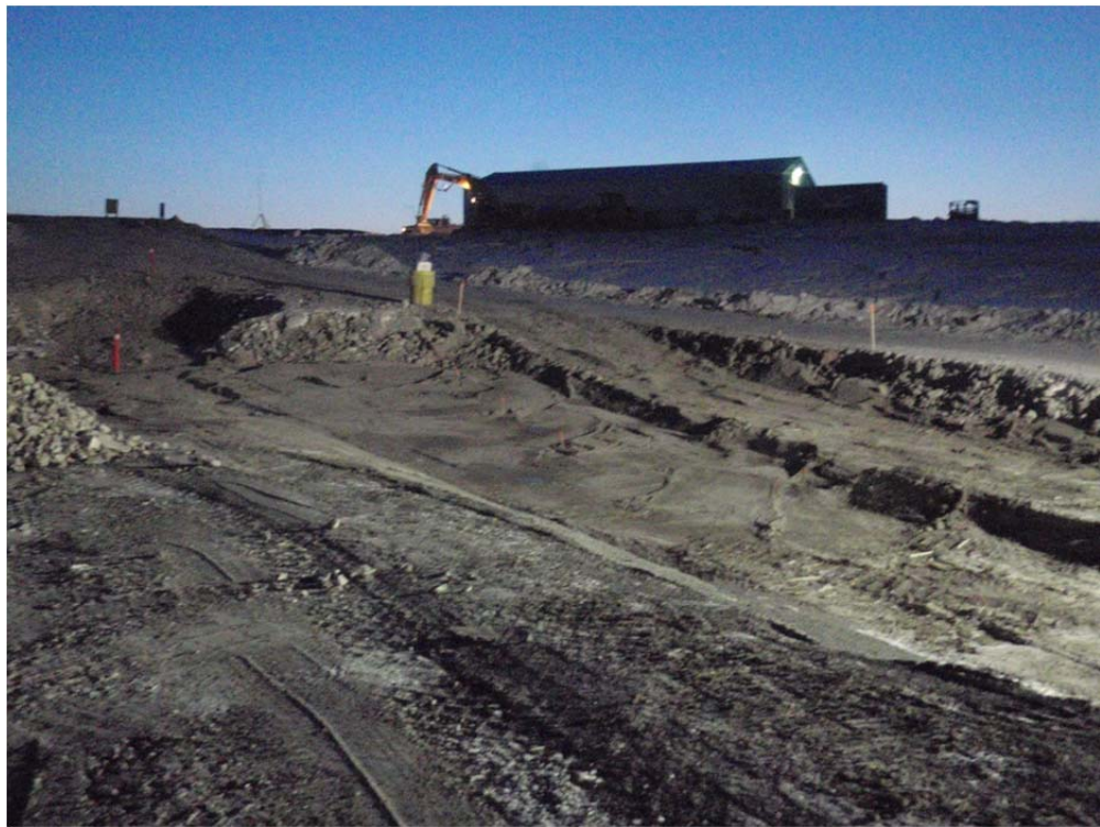
Photo 15: ~NNE view towards the North corner of today's overliner placement. Note that this was the area where a thin skiff of drier crush was placed.
