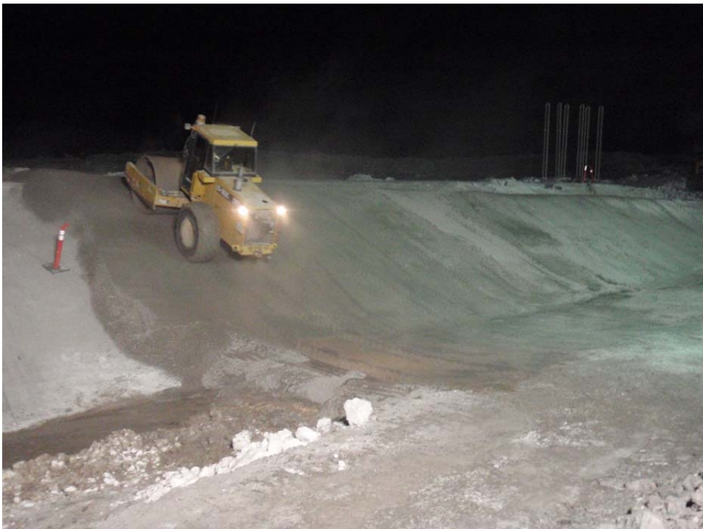
Photo 14: Packer working around station 1+55 on the 2.5HL1V upstream slope.
