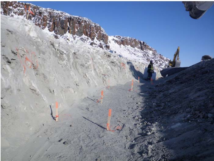
Photo 9: Grade staked placed for bottom bentonite layer on the floor of the key trench for the diversion berm.
