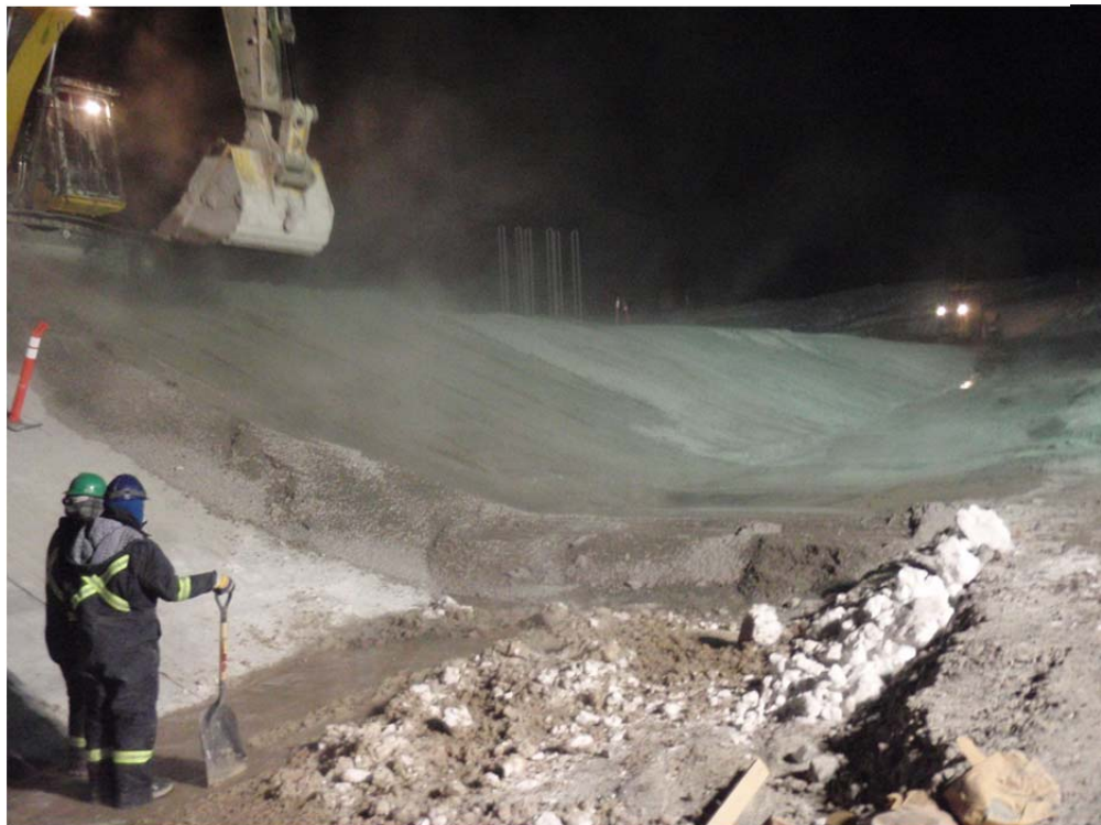
Photo 13: ~ N view of 330 excavator spreading Overliner material around station 1+60. Note bleed water and snow used to slow / trap some of the bleed water.
