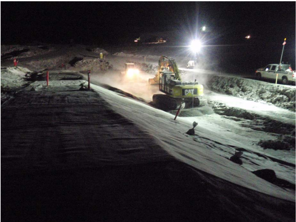
Photo 11: Excavator spreading overliner material around station 1+45, ~NE view.
