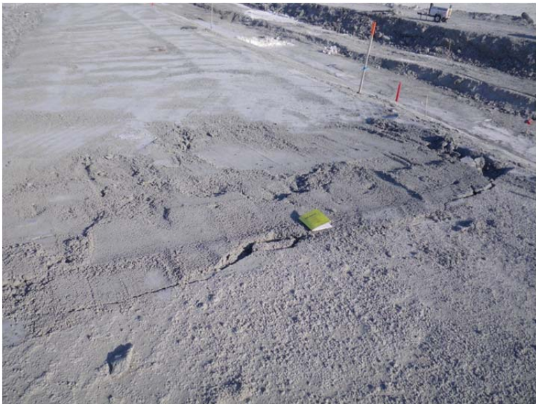
Photo 7: Closer view at the end of the scraped material. As the material was not fully frozen back the surface of the FCM cracked. This cracked material will have to be removed once freeze back is achieved.
